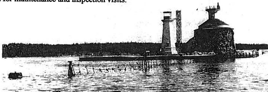
The old tower is demolished as the new tower rises Oct. 3, 1942. Note the anti-submarine nets. National Archives of Canada, PA 105951, Courtesy Allan Ruffman.
